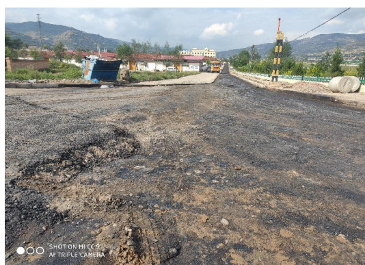
B/F线新农村路面恢复
